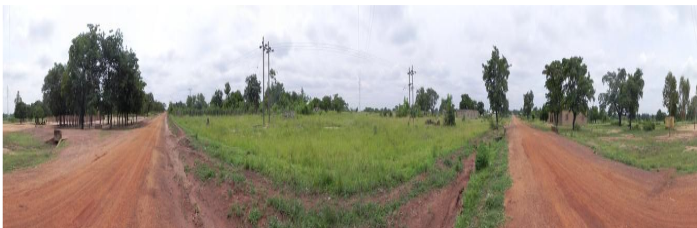
Plate 3: 360°- Panorama at the district road looking south along the MV line for Kaleo PV Site
